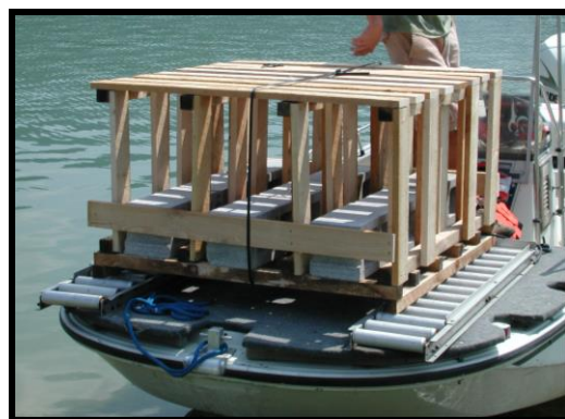
Wooden fish habitat structure built and placed by volunteers with assistance from USACE.
