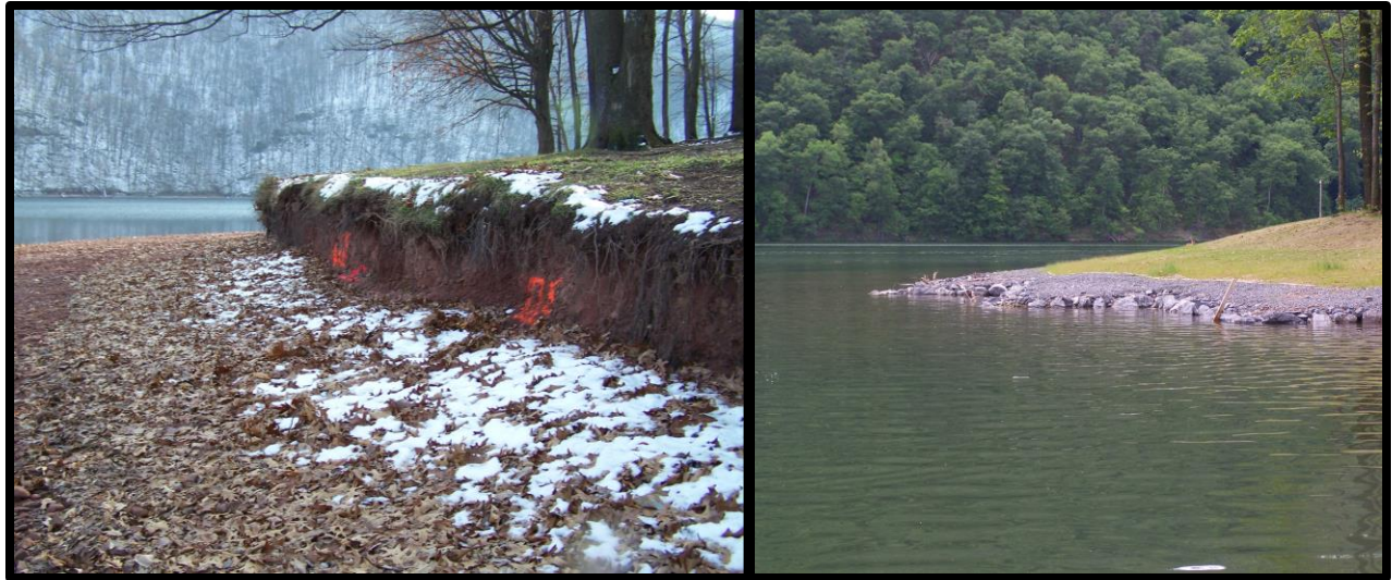
Eroded shoreline at Susquehannock Campground, Raystown Lake before and after stabilization project between PFBC and USACE.
